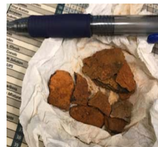
Figure 1 - a very small sample of debris from 2 and half year old VLGC Deck Water Spray system. Total volume of debris cleared after temporary removal of 4 orifice plates could have nearly filled a five gallon bucket. Also cleared from the system were 3- 3inch x 1 inch bolts with nuts on obviously in the piping system since construction.
