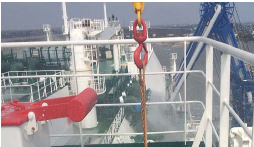
Figure 2 – Deck Water Spray coverage of starboard cargo manifold on a LNG Carrier Photo Credit (Mr. Jamie Wilson, USCG Sector Houston-Galveston)
