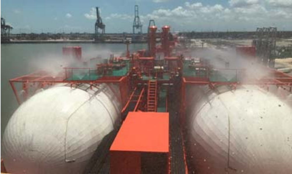
Figure 5 – Excellent deck water spray coverage of deck tanks as viewed from bridge. Good example of why not to only test from the bridge, is there adequate coverage on the other cargo tank tops, manifolds, etc.? Something to think about.
